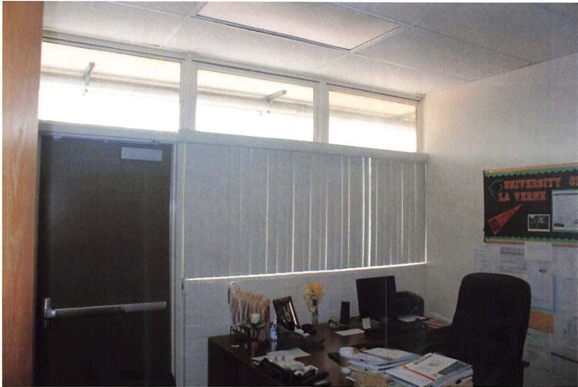
Office – finishes are outdated, needs storage and casework solutions
