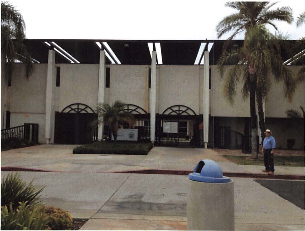
Exterior façade need updating
