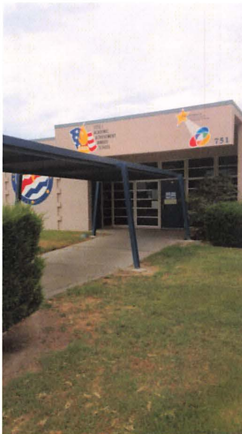
Entry Area needs updating
